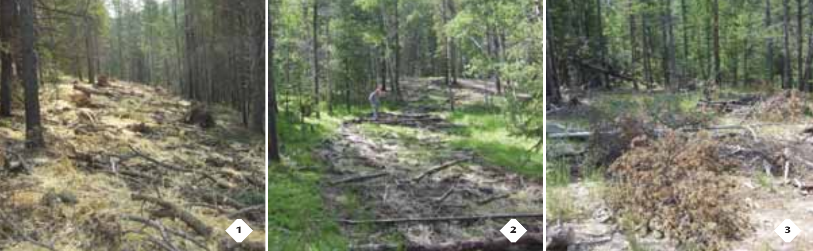
Photo 1: Steps of the Reclamation Process: First, the road or drill site is “recontoured”, during which all fill material is replaced so that the disturbance is at the original natural slope. Topsoil is placed on the top of this. Then, “slash” (dead trees, roots, etc.) is placed on top of the topsoil, in order to hold in soil moisture, prevent the straw mulch and grass seed from blowing away, preclude access by motorized vehicles, and provide nutrients to the soil when it decays. Next the
